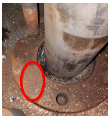
Figure 4. Diagram of the upper packing of the electric valve at the outlet of a steam feed pump.
