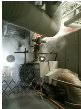
Figure 3. Leakage diagram of the electric valve at the outlet of a steam feed pump.
