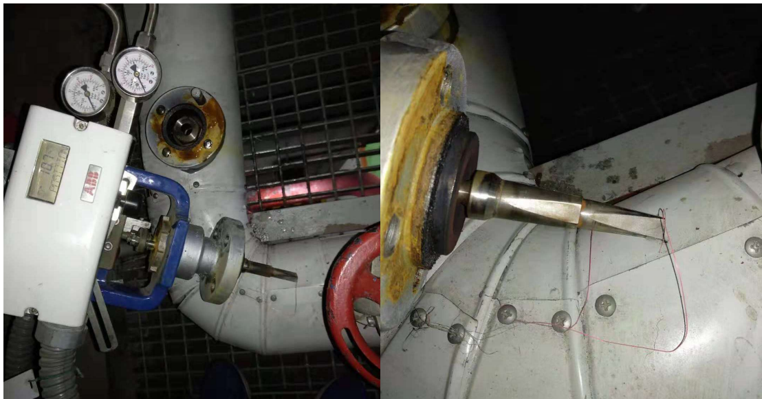
Figure 4. Low pressure shaft seal desuperheated water regulating valve disassembly inspection.
