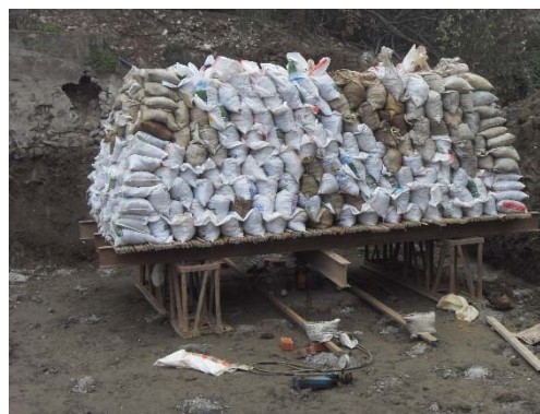
Figure 2. Static load test of CFG pile
