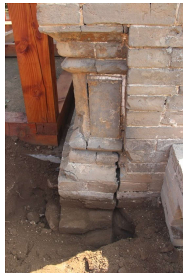
Fig.5 The bottom of Screen the wall is crushed(right)
