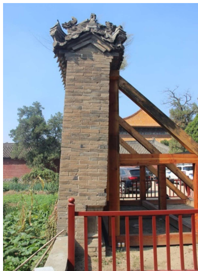
Fig.4 Tilt damage of Screen the wall of Zhong Yue Temple(left)
