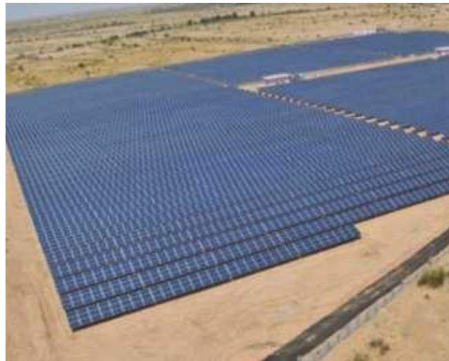
Figure 2: Solar panel installed in Karnataka (Verma, P)
