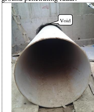
Figure 2. A photo of pipe jacking construction.
