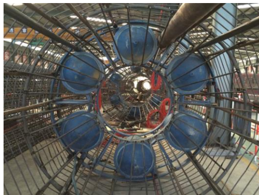
Figure 5. Load cells welded to the steel cage.
