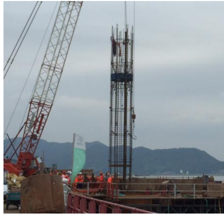
Figure 6. Lowering down of steel cage with load cell.
