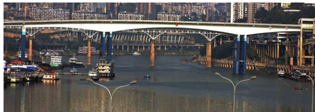
Figure 3 Yuao Light Rail Bridge
