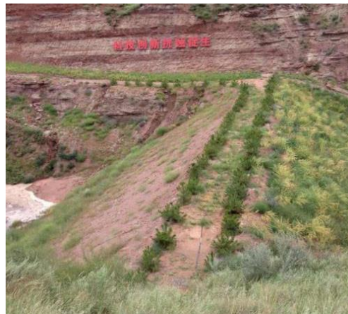
Figure 2. Silt Dam with Modified Materials of Pisha Sandstone
