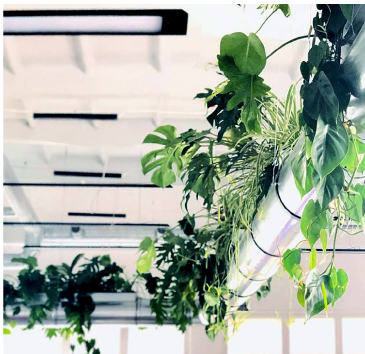
Figure 8. Biofilters mounted in pilot office building in Warsaw.
