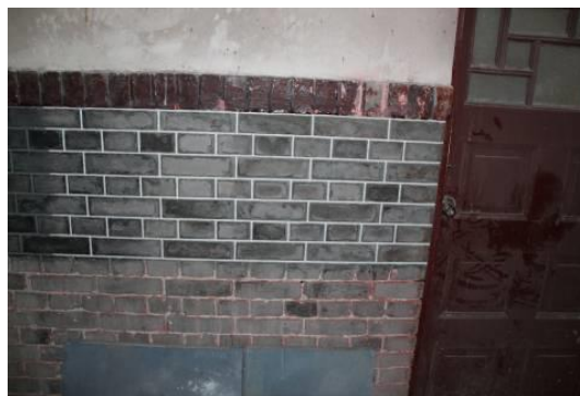
Figure 19. Repaired brick wall surface
