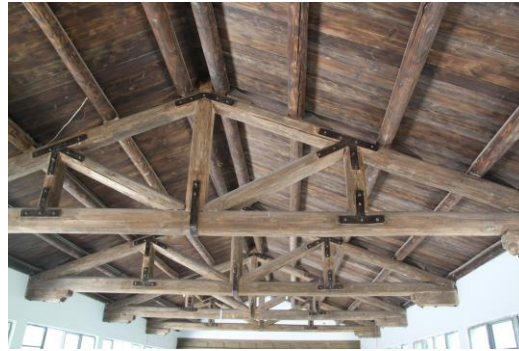
Figure 13. Repair of wooden roof truss of corridor
