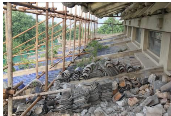
Figure 9. Glazed cylindrical tiles and clay tiles were disassembled
