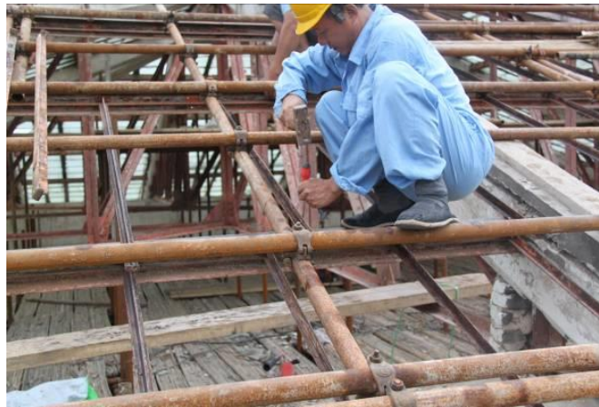
Figure 7. T-shape keels were installed according to original sample
