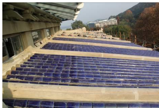
Figure 10. Tiles were paved with cement mortar
