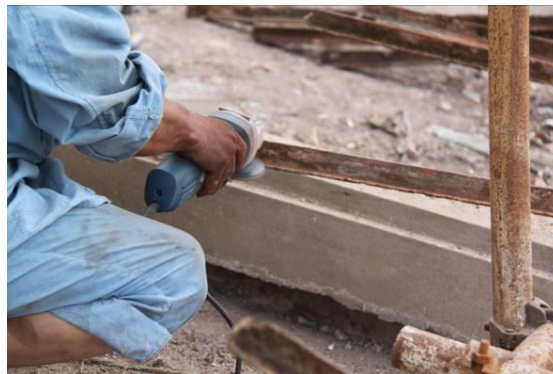
Figure 5. Derusting and polishing of the dismantled iron T-shape keel
