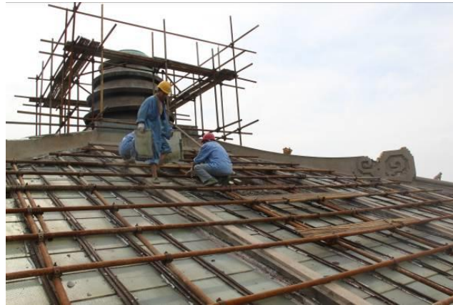
Figure 4. Disassemble glass iron lid strip
