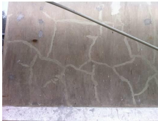
Figure 15. Tiny cracks in wall were repaired
