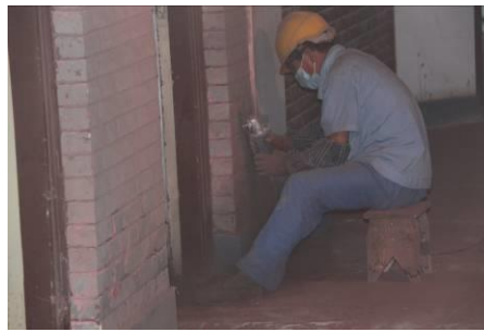
Figure 18. Coatings were removed by polishing
