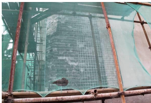
Figure 16. Repaires of cracks at four wall corners
