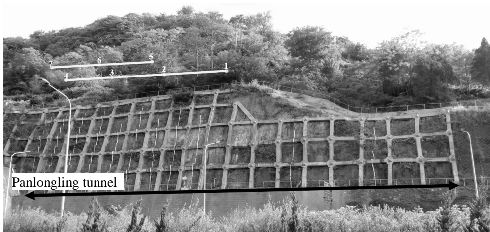
Figure 3. Test Point Layout for K290+400 Slope
