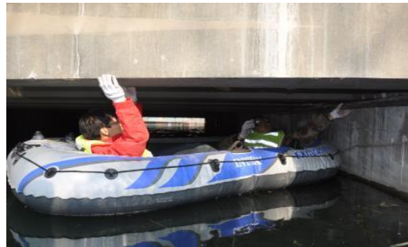
Figure 1. Dewaixi River Bridge
