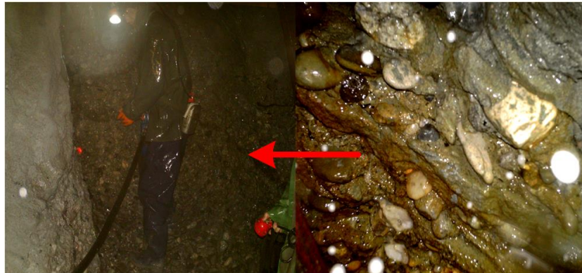
Figure 1. Water-rich surrounding rock in sandy-gravel stratum
