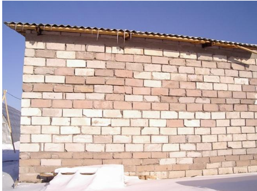
Figure 3. The use of ash-foam concrete in the construction of industrial buildings.
