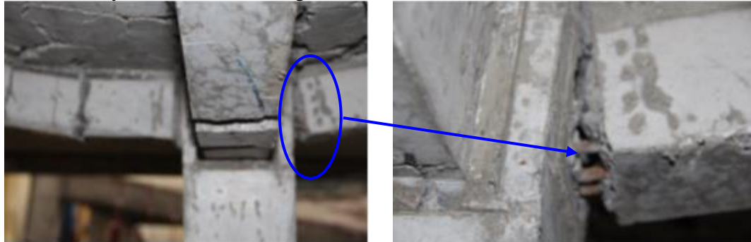
Figure 6. Rupture of steel bar in 2-axis frame beam
