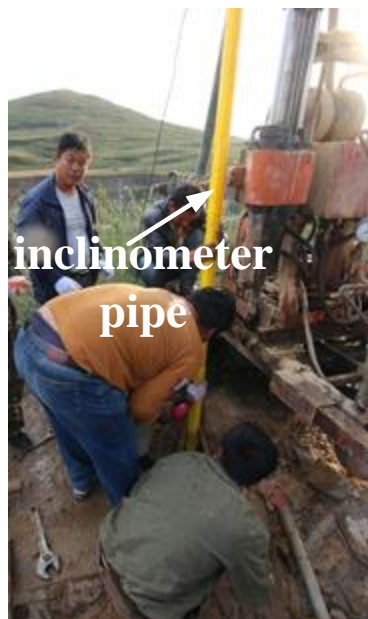
Figure 6. The install of inclinometer pipe
