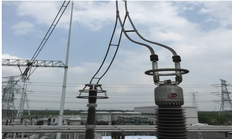
Figure 1 Phase A clamp of the #2 transformer
