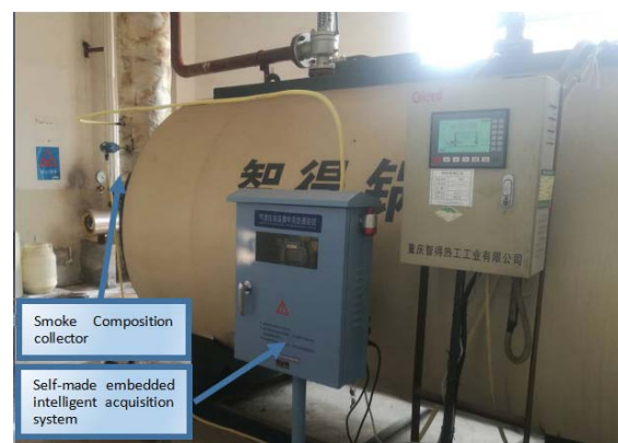
Figure 5. Application example of the intelligent monitoring platform for boilers
