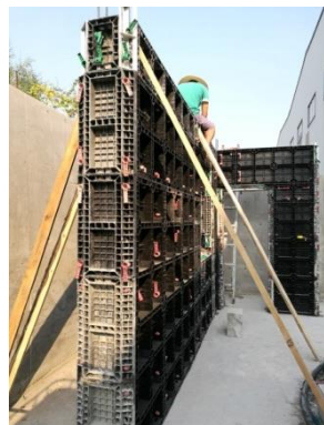
Figure 5. Group 3 supported formwork
