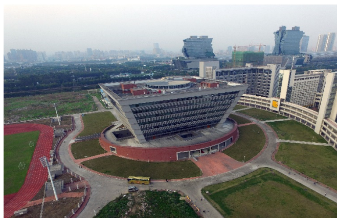
Figure 6 Aerial view of North District (New) library building
