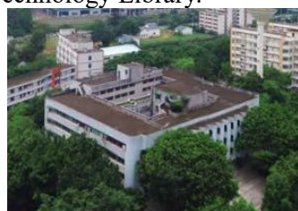
Figure 1 Southern District (Old) Library
