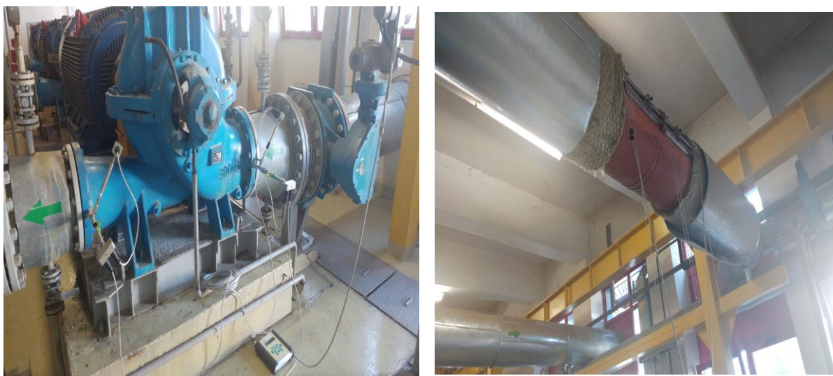
Figure 7. P22F equipment and Fluxus flow rate meter setup for an investigated pump.
