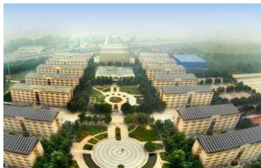
Solar plant of Hebei university of economics and business: all glass vacuum tube collector: 11600m 2 , seasonal tank thermal energy storage: 20000m 3 , design solar fraction: 60%.
