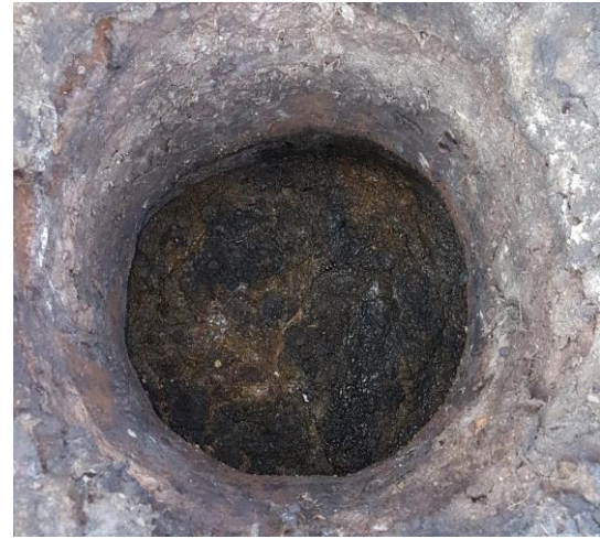
Figure 3. Well with clogged passage.
