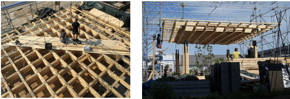
Figure 6. Assembly of the recovered timber lattice-grid roof structure.
