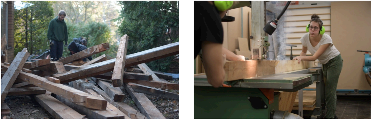
Figure 3. Timber harvested from a demolition site and reworking.
