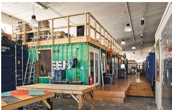
Figure 6 Containers on an insulated plinth in Zone 1
