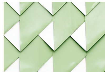
Figure 13. 1:1 mock-up of steel facade from reused sheet metal and dff. [7]
