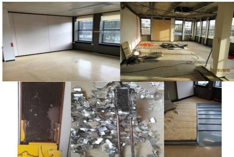
Figure 2. Test deconstruction of a representative unit in the building, from top left to below right corner: View of the office before and after the test. Office door composition. Radiator consisting of aluminium plates and copper bars. Interior wall.
