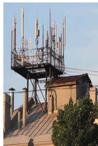
Figure 2. An example of BTS antenna placement on the inclined roof.
