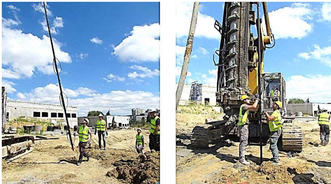
Figure 5. The view of optical sensor in steel, protecting tube during installation process
