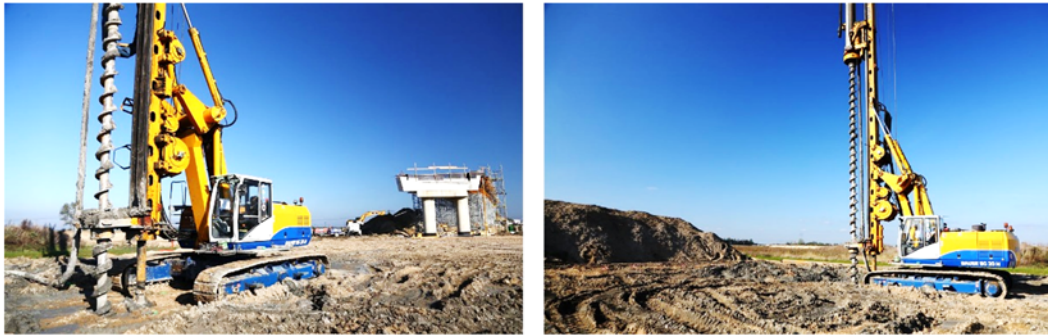
Figure 1. Exemplary execution of Continuous Flight Auger columns on site [Menard archives]
