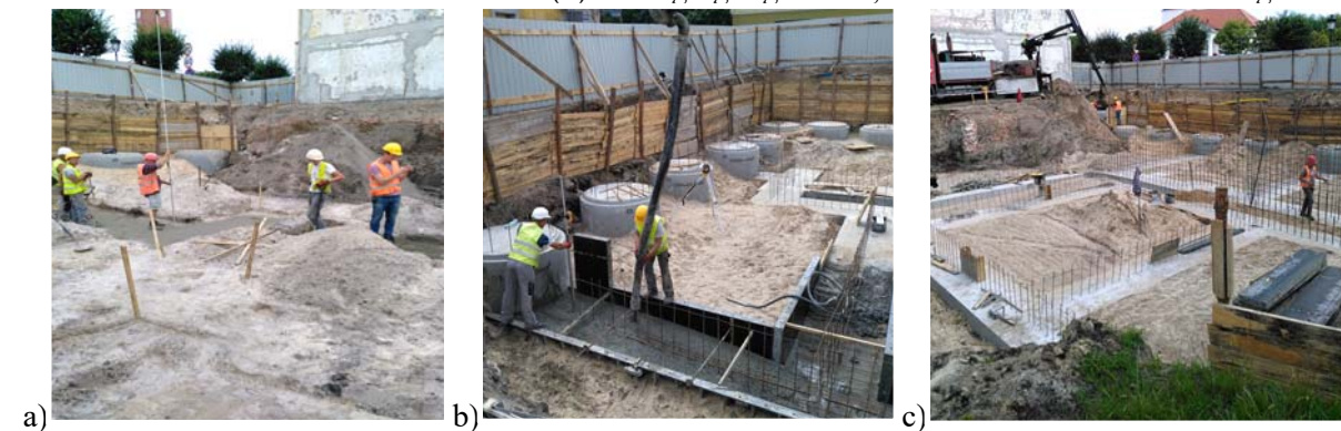
Figure 4. Execution of direct foundations: (a) Laying of continuous footings and execution of B10 concrete underlay (b) Laying formwork of continuous footings and concreting (c) Stripping and covering foundation
