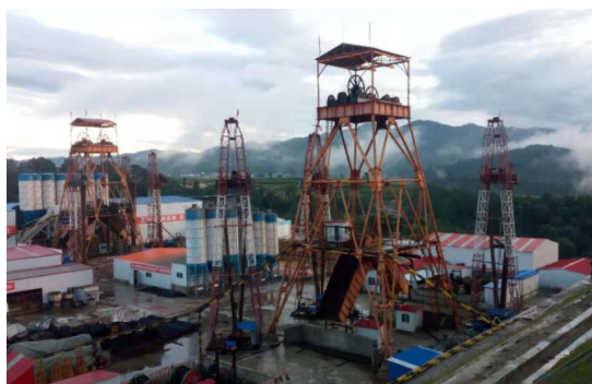
Fig 7. The photographs of sinking head-frames and grouting boring towers of main and auxiliary shafts of No.2 vertical shaft
