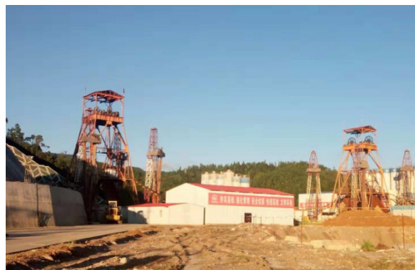
Fig 7. The photographs of sinking head-frames and grouting boring towers of main and auxiliary shafts of No.2 vertical shaft
