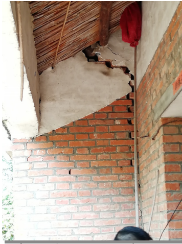
Figure 3. Structure damage near the left wooden beam
