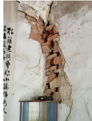
Figure 4. Damage on the top of the right wall
