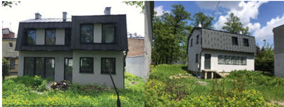
Figure 1. Improperly designed new building. a. northern façade – fully glazed, b. south-western façade without glazing [by EJ Sobczyk].
