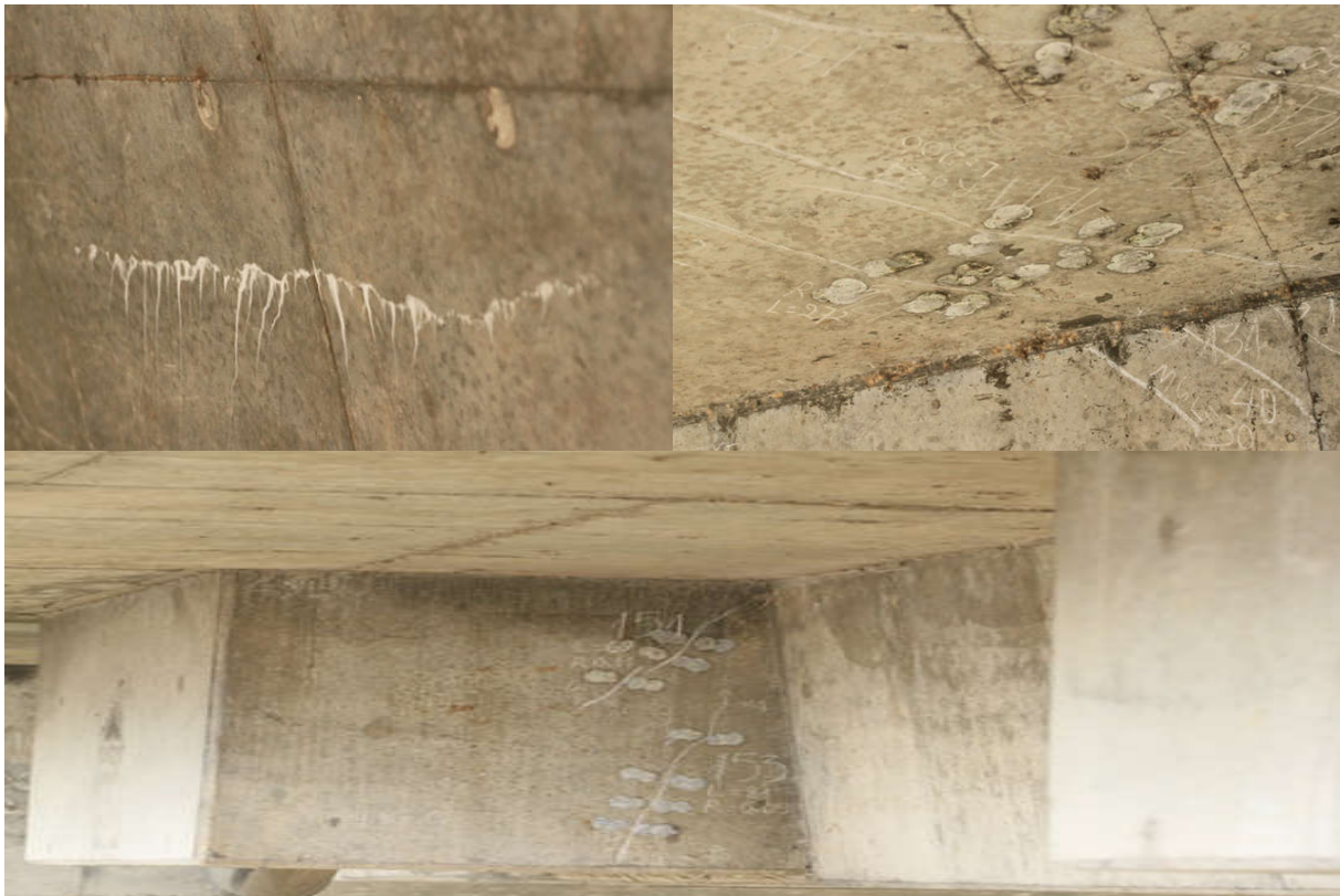
Figure 2. Cracks of bridge support elements.
