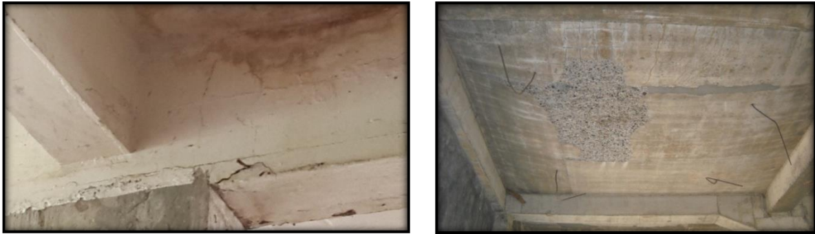
Figure 1. The damages of (a) the beam and (b) the slab on the existing building
