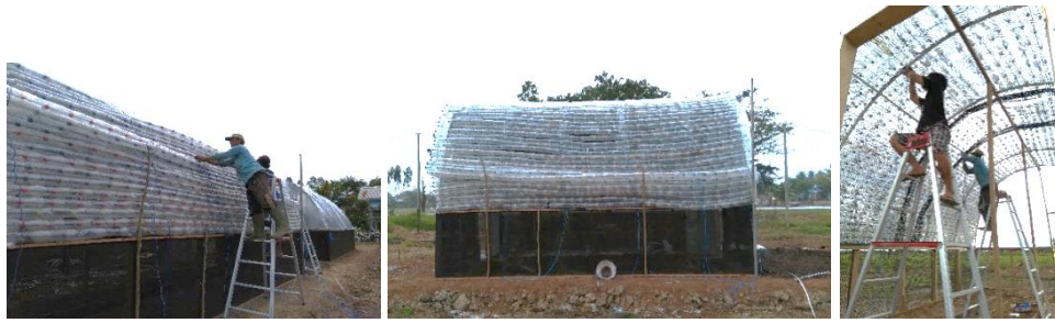
Figure 2. Greenhouse with used bottle roof cover material
