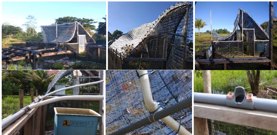
Figure 3. The roof structure material of the PCV pipe is unable to withstand wind loads
