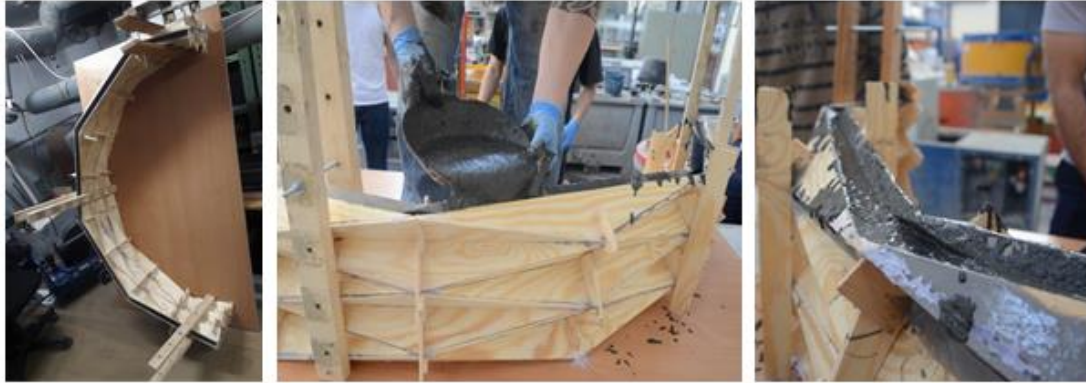
Figure 11. Concreting the origami arch.
