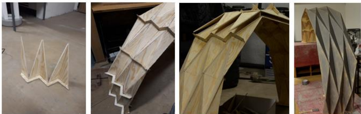
Figure 10. Building the formwork.
