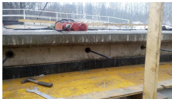
Figure 7. Transverse prestressing
