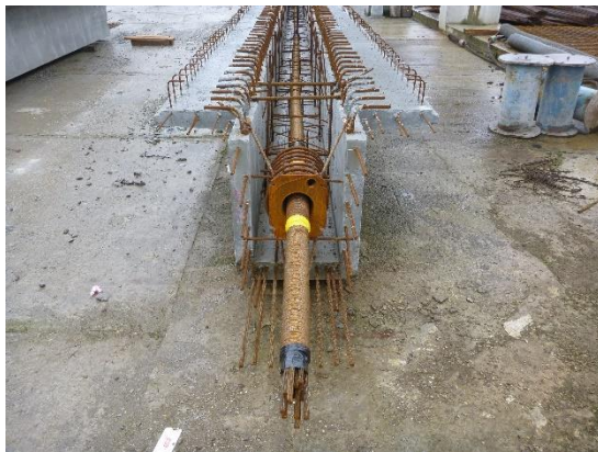
Figure 1. Complete \Omega beam
