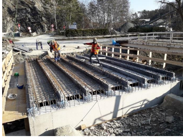
Figure 9. Assembled beams on site
