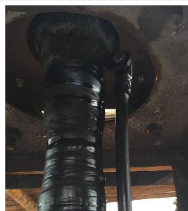
Figure 3. No fixed ground wire connected to the grounding copper block.
