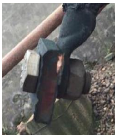
Figure 2. No fastened connection bolts.
