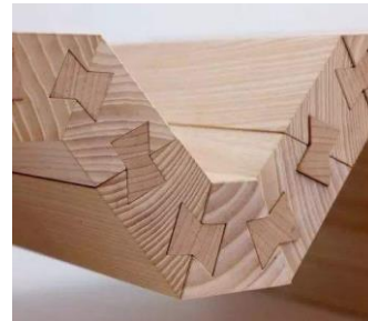
pic.2 dovetail tenon
