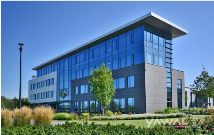
Figure 1. Fragment of the facade using the stay-and-cross-beam system. YAWAL FA 50N HI (Poland)
