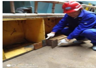
Figure 2 Channel fixing
