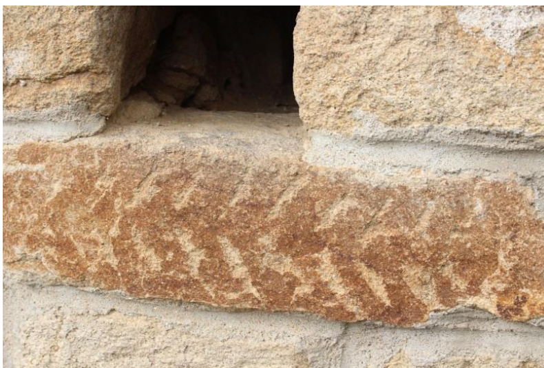
Figure 5. A detail of the rocky masonry with a venting hole.
