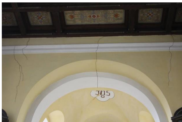
Figure 7. Cracks in the vault of the triumphal arch.
