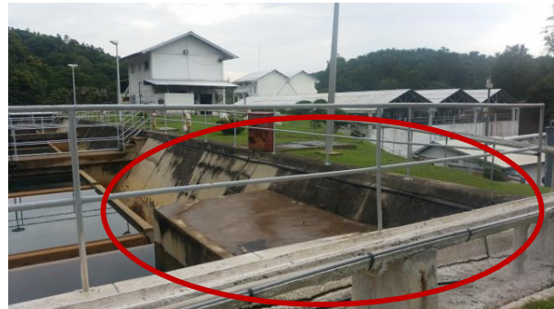
Figure 2. A structural crack was observed on the Water Sedimentation Plant storage tanks.
