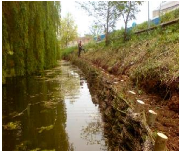
Figure 4. Installing stakes to protect the river bank form erosion
