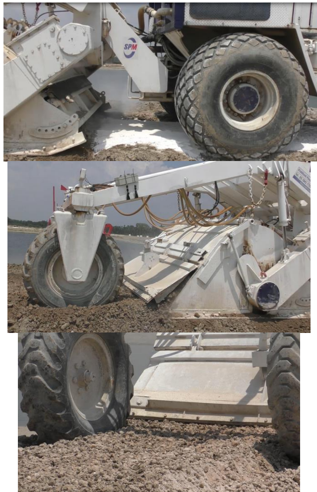
Figure 9. Insitu Stabilisation of Marine Clay with 4% Lime
