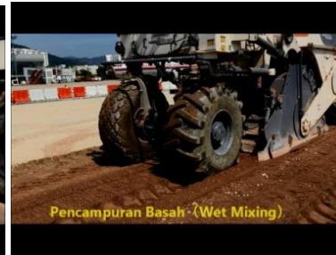
Figure 2(b)(ii) Wet Mixing
