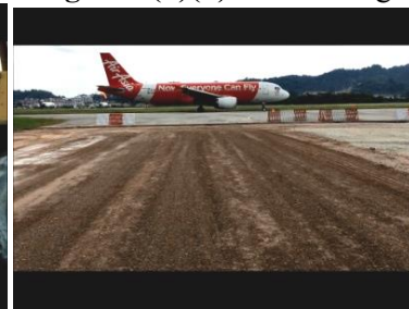
Figure 2(c)(ii) Finished Layer of Stabilized Base
