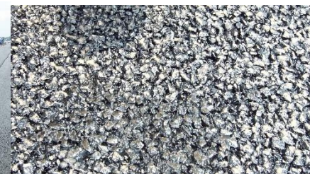
Plate 5 The surface of porous asphalt
