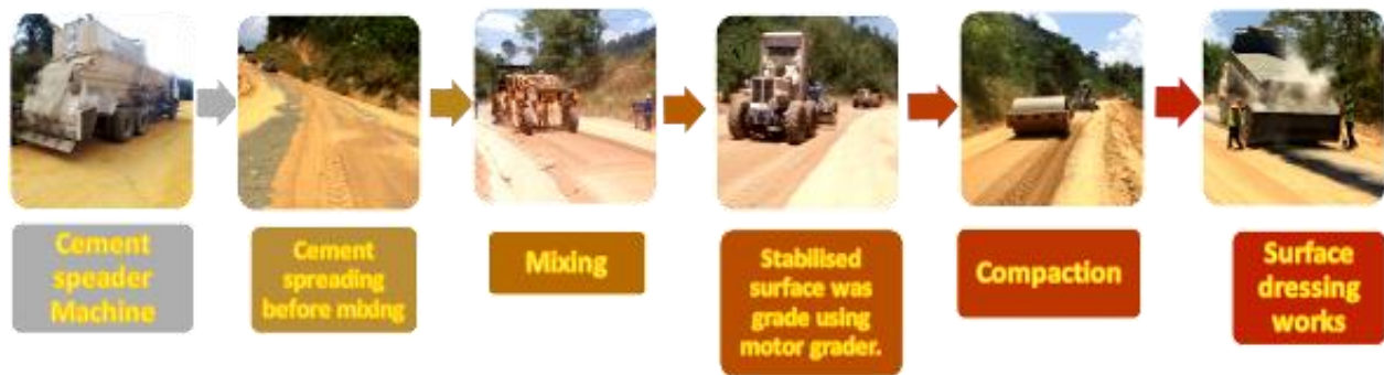
Figure 7. Soil stabilisation process.
