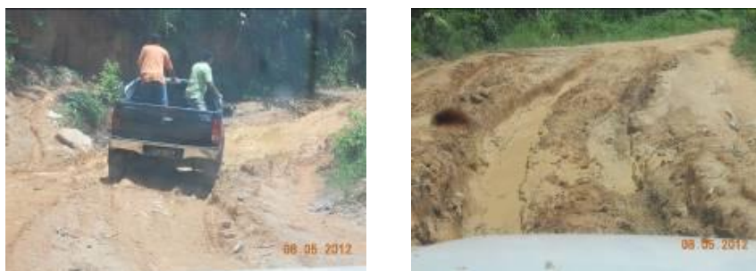
Figure 1. The condition of an existing road before construction.
