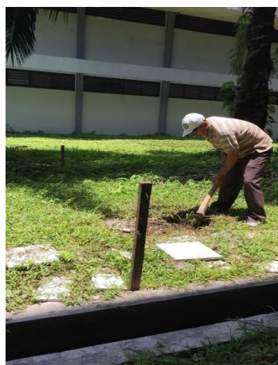
Figure 4. The process of digging soil and bowplank work
